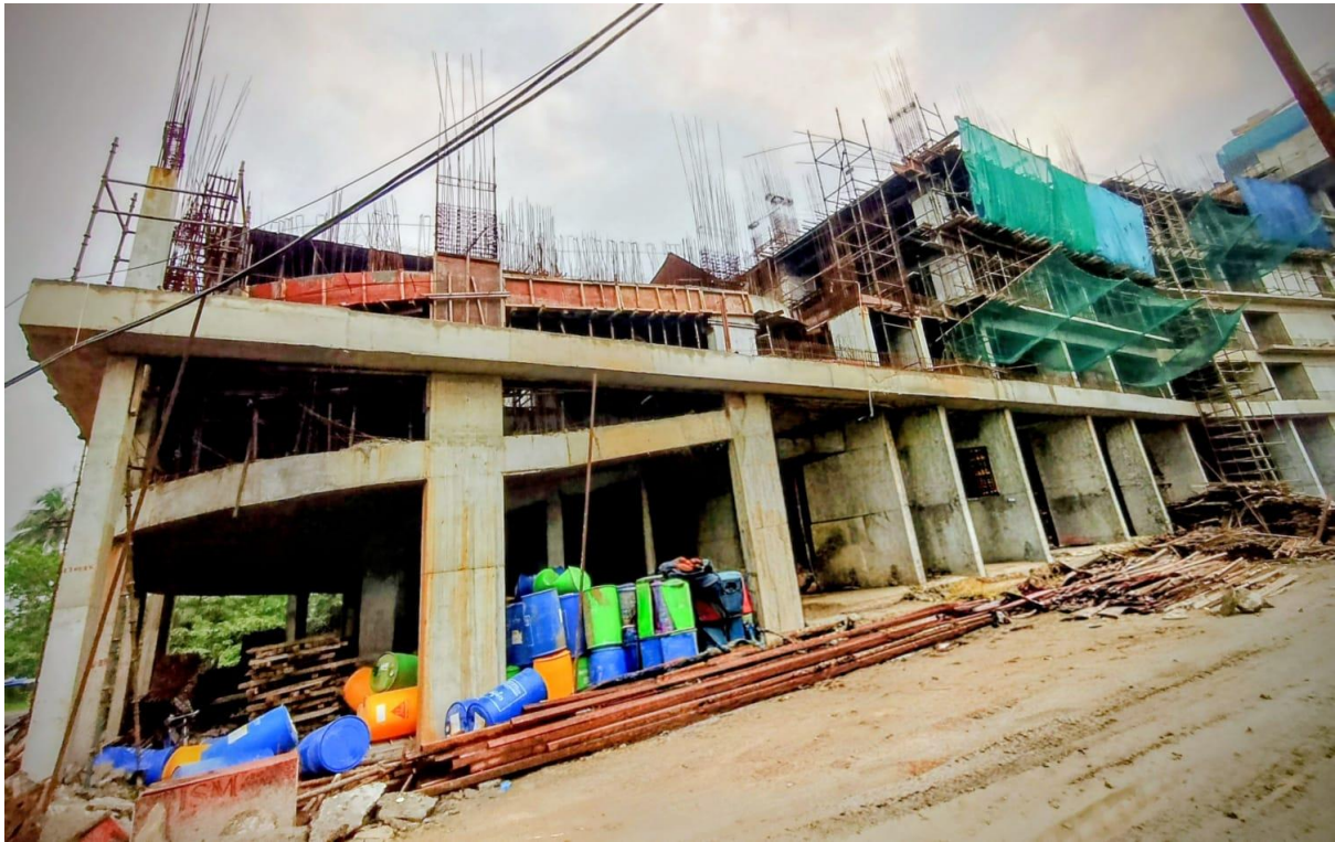
Tower 16 – Super-structure work in progress i.e. 5 th slab work in progress.
